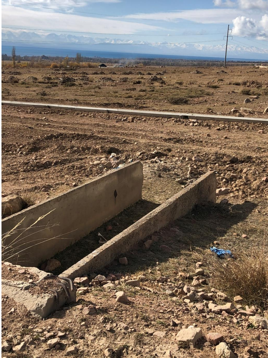
Juxtaposition of Old Derelict Canal and New Canal that Carries Water from the Refurbished Reservoir
