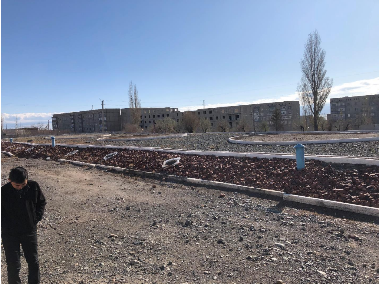
First Potable Water Reservoir (Underground)
