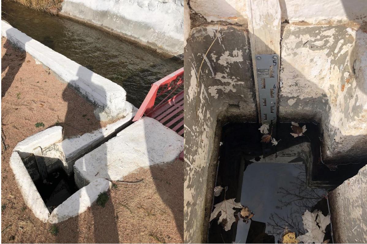
Staff Gage for Measuring Flow in the Canal
