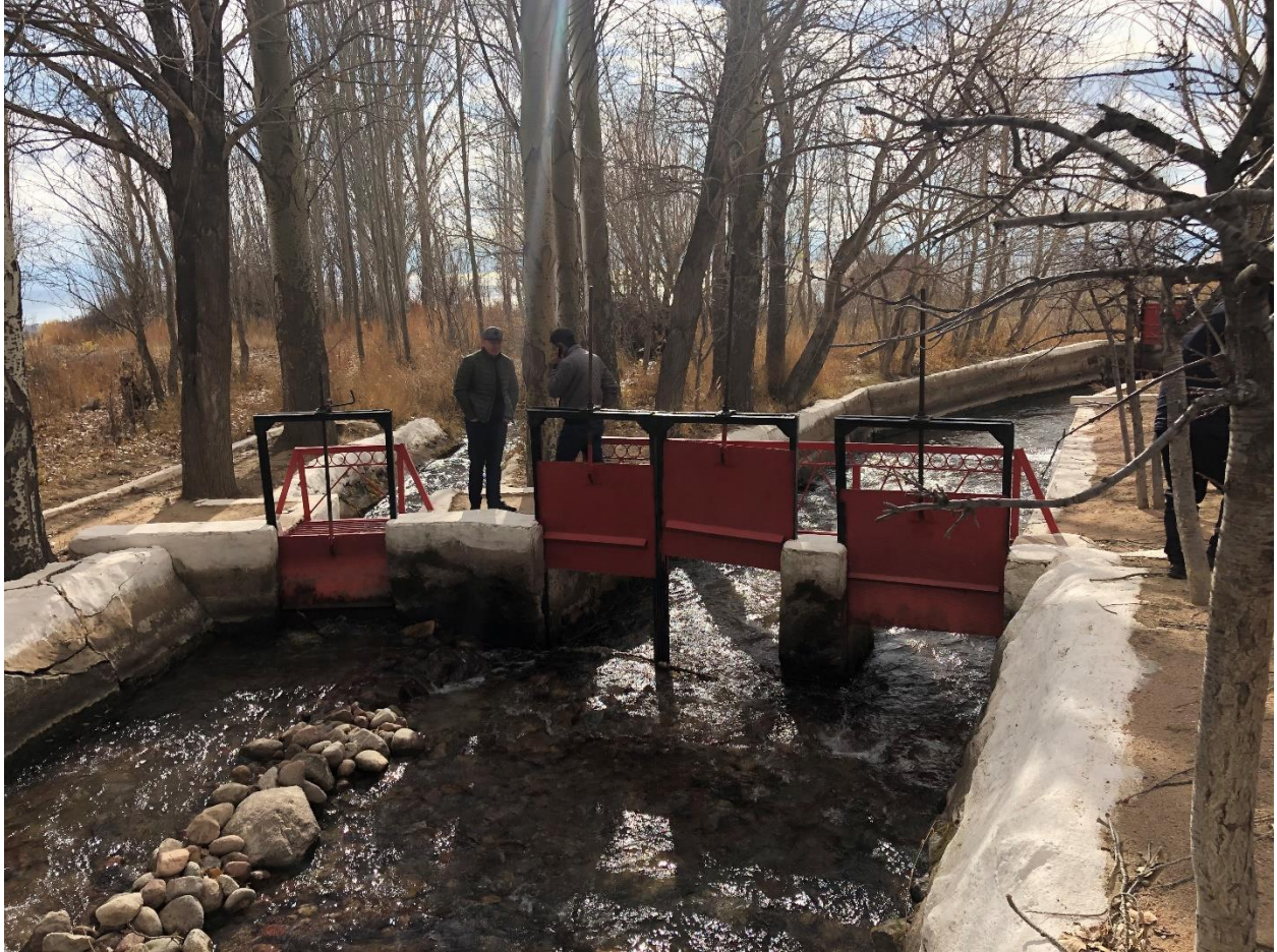
Diversion Structure that Splits Flow Between Cholpon-Ata (left), Which Treats the Water and Delivers it for Household Use, and the Irrigation Reservoir (right).
