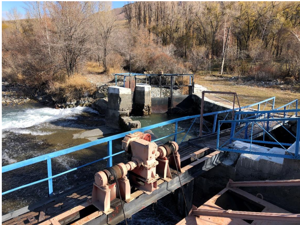
Gate on the Right Bank Canal at the Diversion
