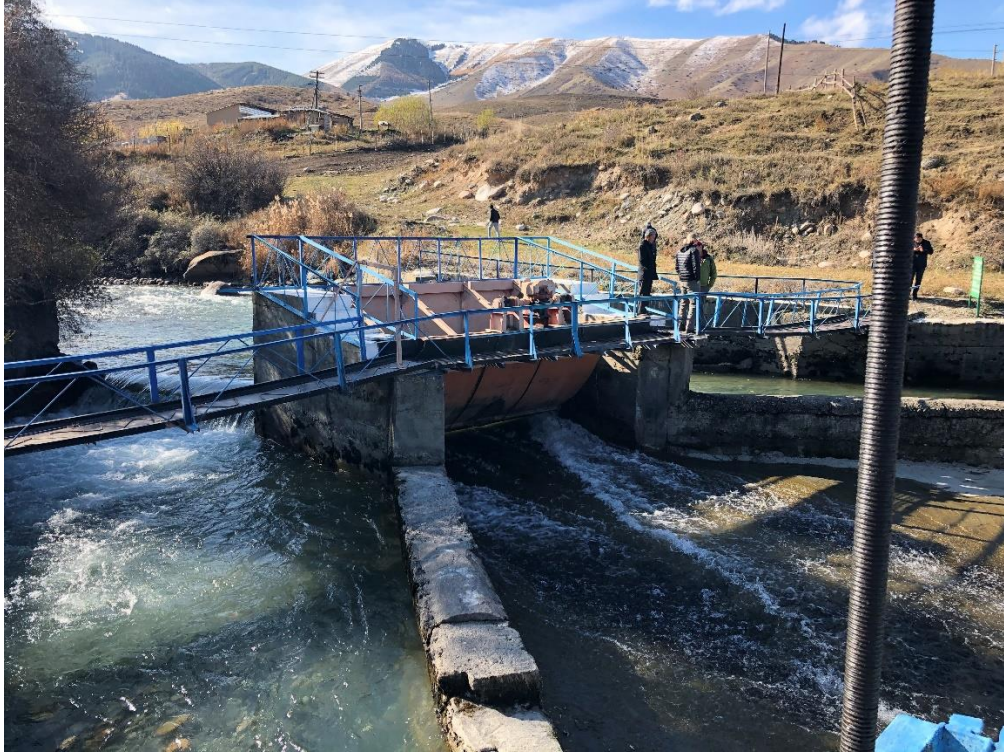
Looking Upstream at the Irrigation Diversion on the Ak-Suu River
