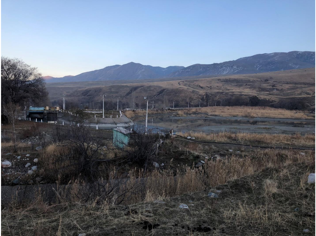
Dam with significant sedimentation on the Ala Archa River
