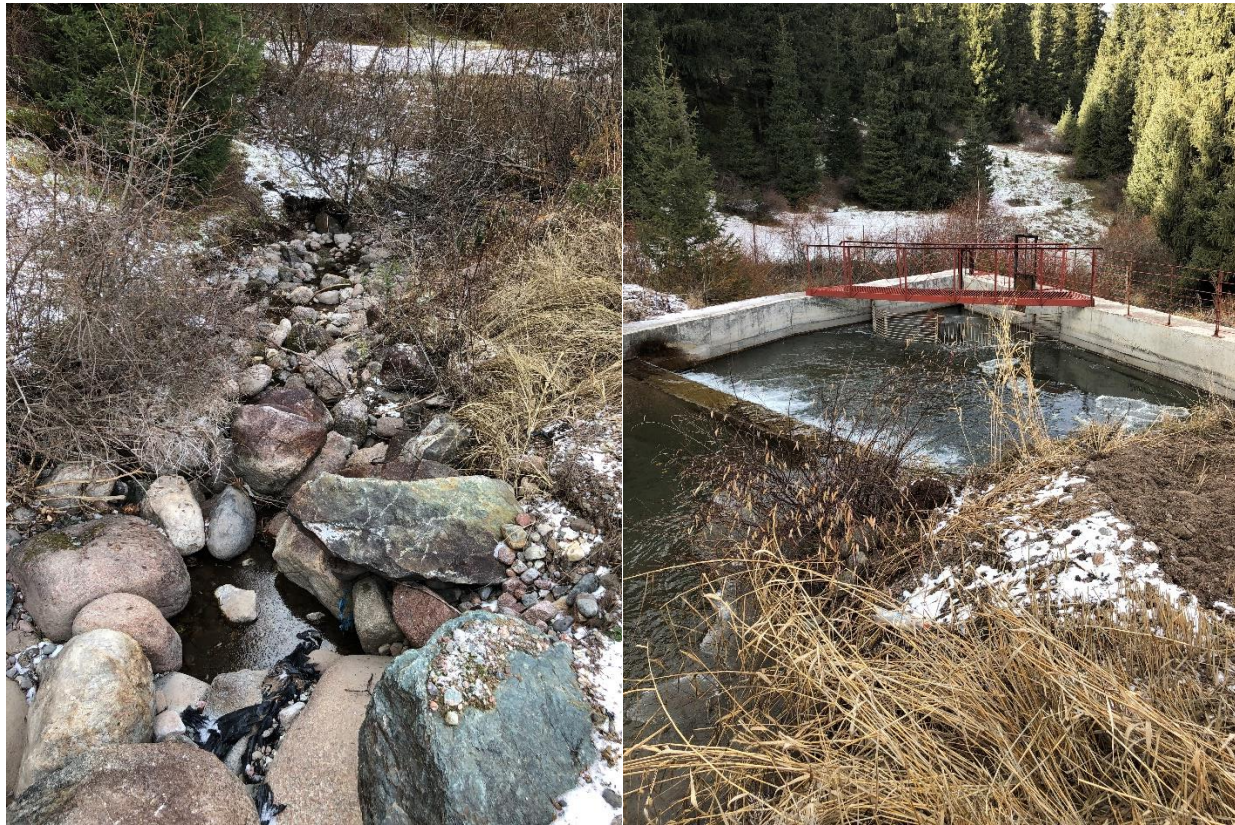
Dewatered Channel (L) and Settling Basin (R)
