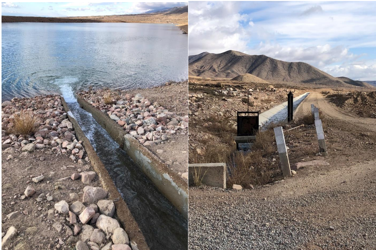
Concrete Canals Filling the Reservoir
