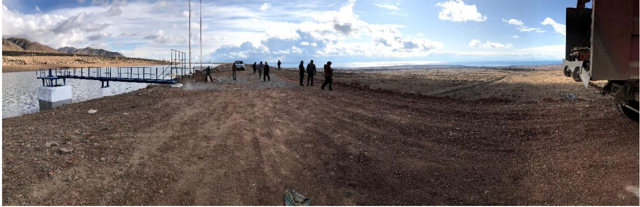
Photo Along Dam Crest Showing Outlet Works and Delivery Canal
